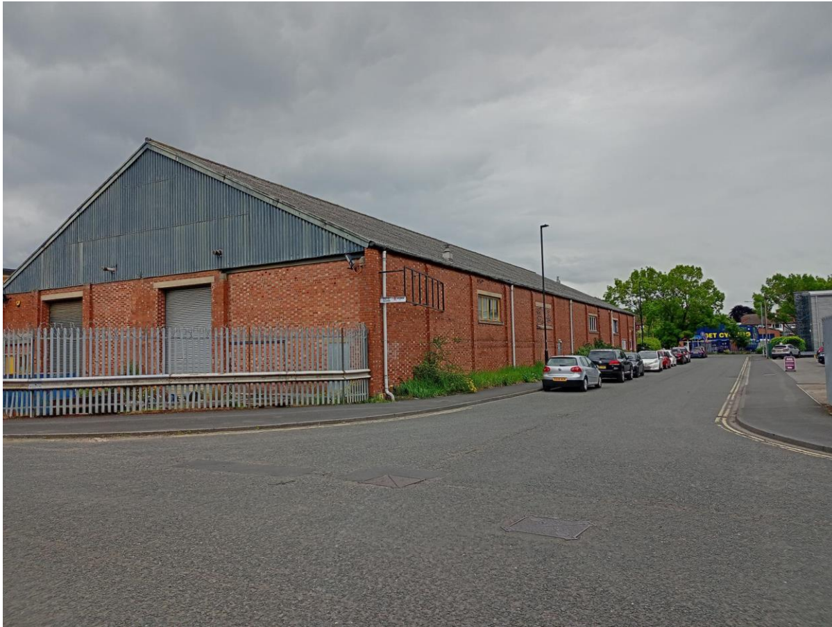
Warehouse on south side of the site
